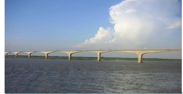
2 Lane Bridge over river Brahmaputra, Assam
